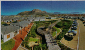
WORLD-CLASS: Aerial view of the boardwalk at Evergreen Muizenberg, which won an award from the Timber Frame Builders' Association earlier this year.
